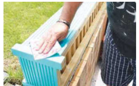
The base coat is de-nibbed with a fine abrasive and dusted off
